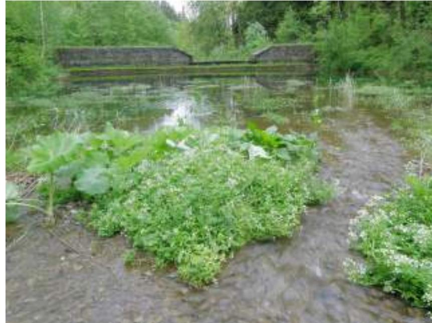
*Retention constructions to hold floating materials at Bohdašinský Stream and Kamenický stream (Rychnov Region); during minimum flow rate retention constructions might provide for survival of water organisms.*
